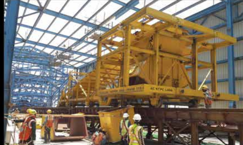
Erection and Alignment of Material Handling Equipments
