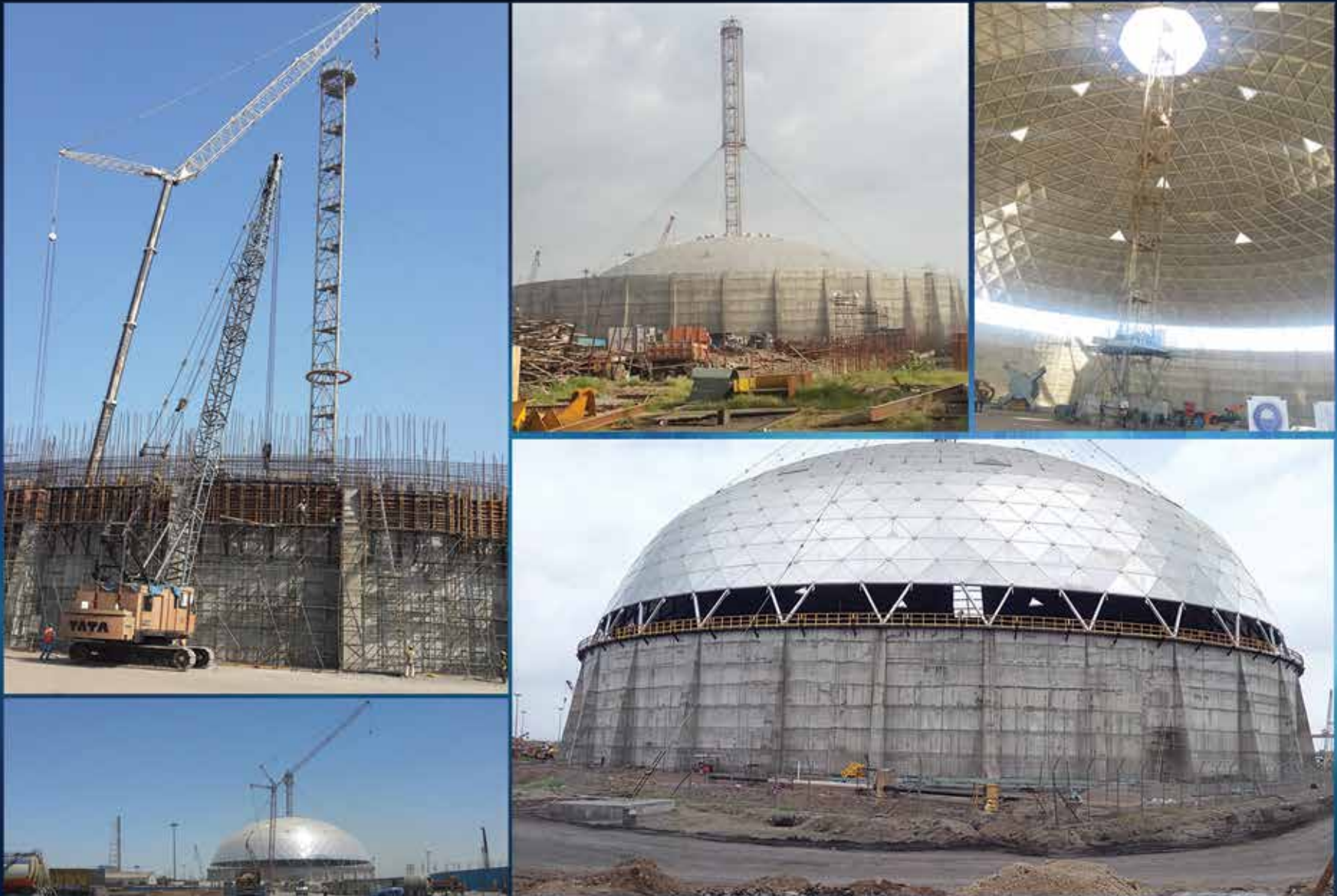
110 mtr Dia DOME for Gasification Plant, Reliance Refinery, Gujrat, India
