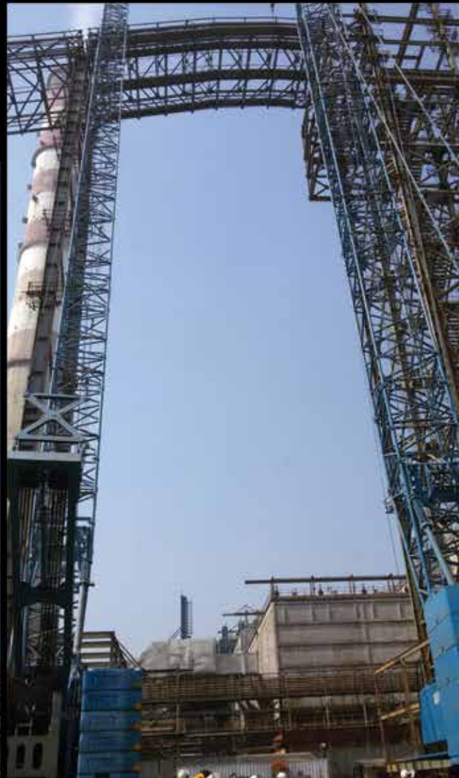
Erection of Gallery at 85 mtrs height, OPGCL-Odisha
