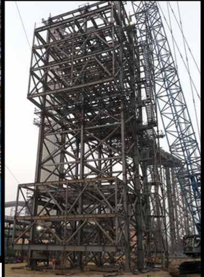
Erection of Gallery at 85 mtrs height, OPGCL-Odisha
